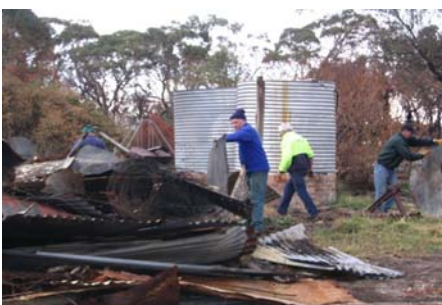
Removing fire damaged materials
