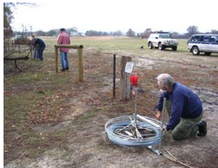
Rebuilding fire damaged fencing near The Grampians
