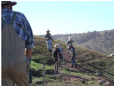
Installing new fencing out of Licola
